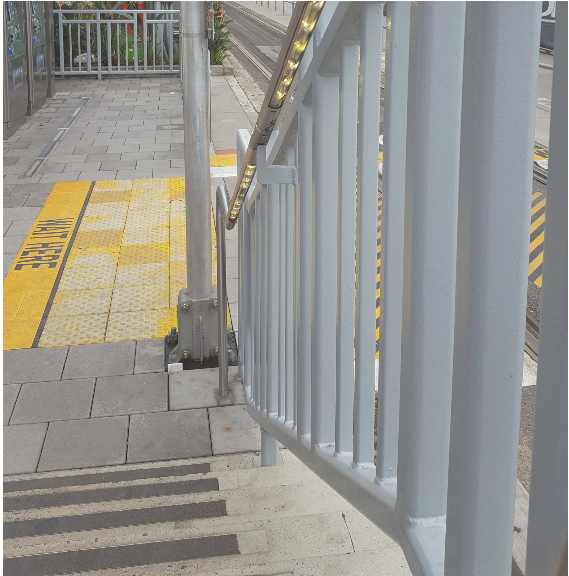
New LED lights on the stairs at Pico Station to warn riders that a train is approaching. Photo by Anna Chen/Metro.
