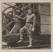
HE HANDLES weighty matters of HE HANDLES weighty matters of the Los Angeles Railway, often 25 tons at a time. He is C. J. Simmons of the maintenance of way department, in charge of the big crane at the Vernon yards. The hoist is used extensively at the yards in stacking ties and rails and lifts big loads in general track construction.
