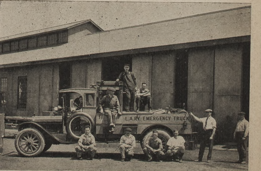
Grouped Around the Speedy Emergency Truck, the Men of the Company Garage Are Looking Handsome With the Garage Building For Background.
