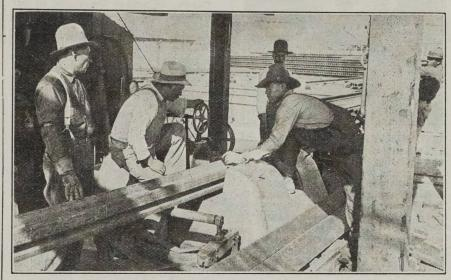
SHAPING the rail for various sized curves and pieces of special work is a feature of track construction that keeps a group of men busy at the Vernon Yards. Before a piece of spe-cial work is installed a dress rehearsal is held in which the rails are fitted to-gether as they will be in the street and measured to fractions of inches.
