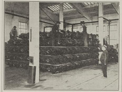
inghouse type motors which are to be used in four-motor equipment on new cars and in converting some of the present two-motor cars, were received at South Park shop last Tuesday, and stored. The 96 motors made three car-loads. One of the derricks was run from the Vernon yards to the shops
