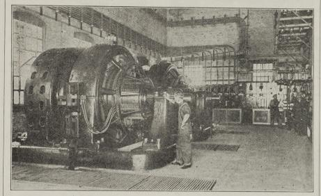
THE picture above is an interior view of the Sentous substation on the Division 4 property, showing the two big 1,000 kilowat motor generator sets, which are now being augmented by the installation of a 1,500 kilowat rotary converter. Although the new piece of equipment is fifty percent
