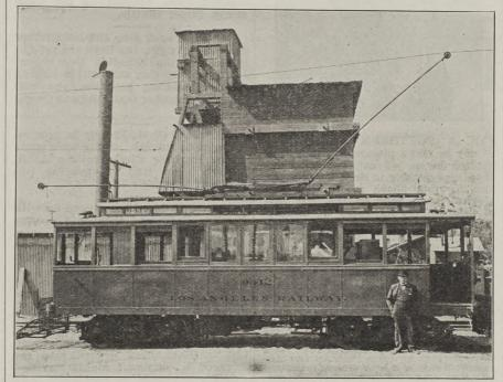
A new sand car pictured above, capable of carrying 12 tons of sand has been rebuilt at the main shops and carries number 9412. It is painted in green of maintenance and way equipment.
