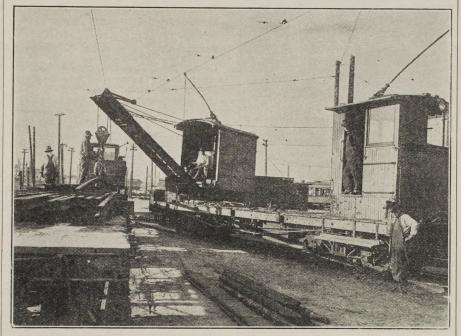
MAINTENANCE OF WAY car 9225 is not the biggest hoist owned by the company, but around the Vernon Yard it is quite "some pumpkins" when rail has to be moved on and off flat cars for track department work. flat cars for track department work. In the Vernon Yard it is frequently necessary to put down temporary track for a special job and remove it in a comparatively short time. This makes the work of the crews on the maintenance of way cars particularly reacting.
