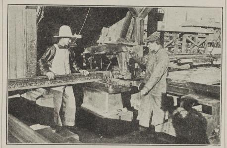
SPECIAL work, such as curves, switches and cross-overs are laid out in the Vernon Yards according to exact measure. Then the steel rail is taken out to the place where it is to be laid, and put in with a minimum of delay. Pieces of straight rail are of delay. Pieces of straight rail are cut to the required length before leaving the vard on a power saw, shown
