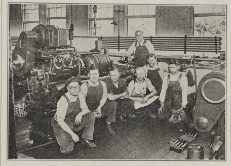
HE lathe shown in the above picture is one of the latest pieces of machinery installed at the South Park shops. It is technically designated as a 12-speed 20inch American lathe and is used for general shop work.
