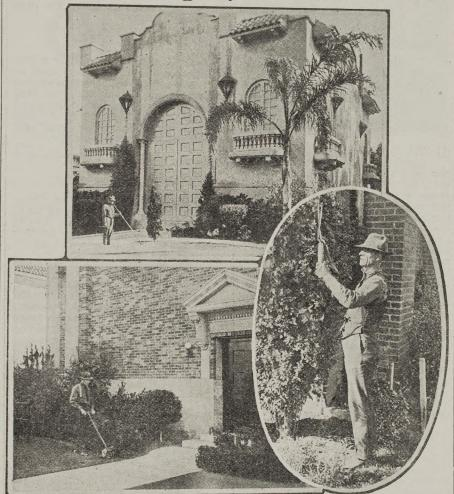
THE noiseless, automatic substations that have been built by the Los that have been built by the Los Angeles Railway in recent years, have proved to be improvements to the appearance of the districts in which they have been placed. In addition to employing artistic architecture to house the electrical equipment, the company has surrounded the buildings with lawns, shrubs, and flowers, that would be a credit to a pretentious residence.
