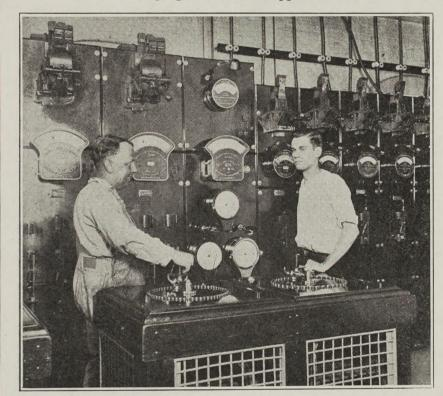
HE flickering fingers of delicate electrical meters shown in the background of the photo above indicate the load conditions on the lines fed by the main substation at Sixteenth and San Pedro, where this picture was taken. A blockade, followed by a sudden clearing, so that a dozen motormen are winding up con-trollers at the same moment, is im-
