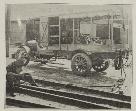
O keep the points of special work which are subject to particularly hard wear up to the copper track level and to build up "cupped" rails, the track department uses the Lincoln portable welder shown in the picture The complete welding apparatus is mounted on a truck. The current is taken from the trolley wire, and runs through the generator that can be seen on the truck. The metal weight
