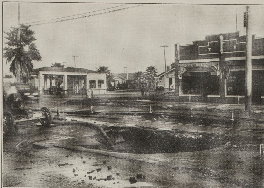
The above cut shows what happened to the Los Angeles Railway car tracks when a 12-foot water main on West 54th Street burst about 100 feet west of Western Avenue on September 10, 1926. The car tracks were out of service for eight hours, which was the time required for repairs to the water main and the car tracks.
