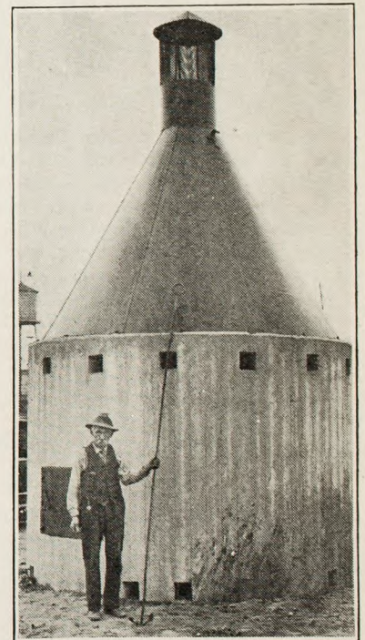
John Dempsey, Engineer of the New Incinerator at Vernon Yard
