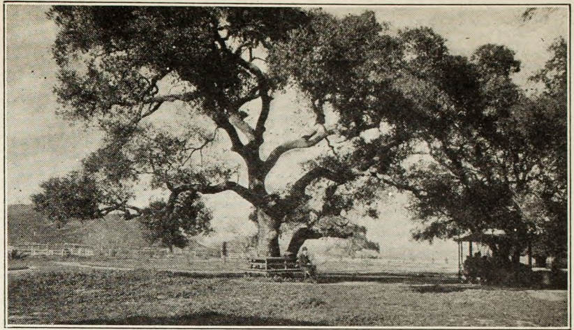
This beautiful old oak stood on the site of the Los Angeles Ostrich Farm. At the right of the picture is the waiting station of the Ostrich Farm Railway in 1887. Today this tree stands on the site of the present Griffith Park Playground.
