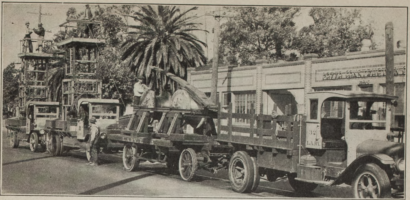
Tower crews with trucks and reel trailer, making replacements at Macy and Alameda Streets. On top of rear truck, left to right: Charles Colen and Lawrence Leusch, Linemen; C. G. Woelker is the driver of the rear truck, though he is hard to see in the picture, as are W. T. Smith and Julius Linares, drivers respectively of the middle and front trucks; R. E. Baker is atop of the tower on the right; James Whitehouse is on the ground, flagging; Leo Maag, Lineman, has his hands on the wire reel.
