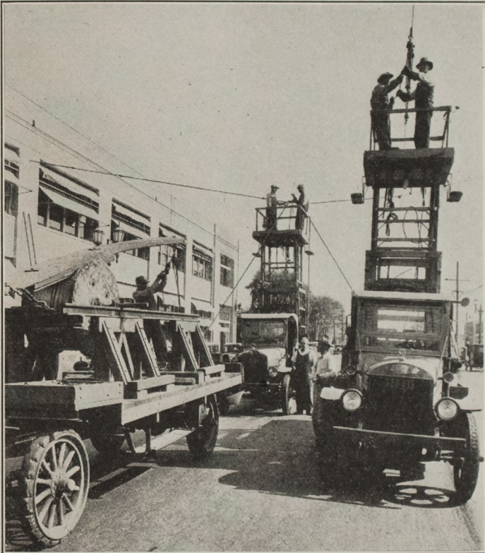
STRINGING TROLLEY WIRE, SOUTH MAIN ST.
