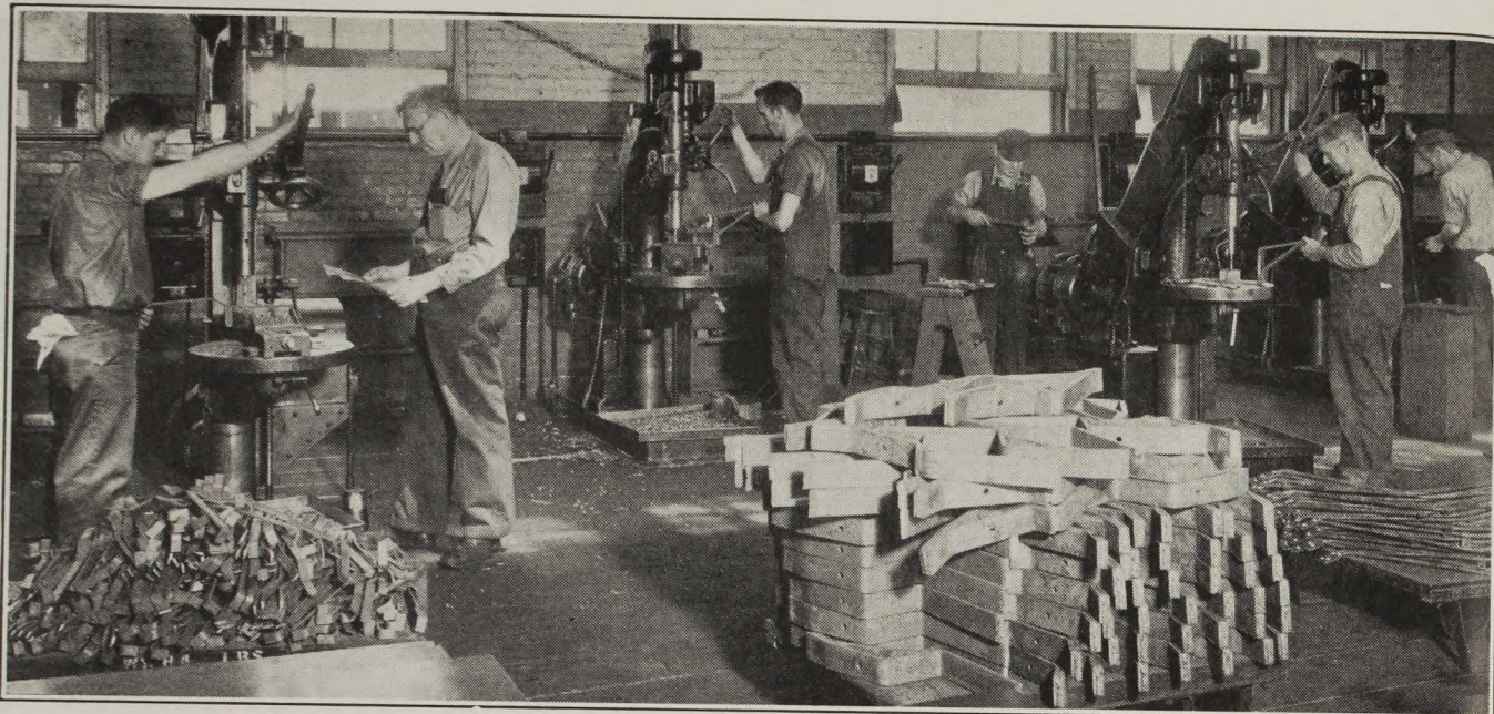
A part of the drill-press room at the South Park Shops commencing to drill a small portion of the 100's of miscellaneous brackets, braces, panels, etc., that will be required for the reconstruction of 53 type "H" cars to type "H-4." Left to Right: C. L. Lock, M. E. McCune, Foreman; W. V. Cook, George S. S. Lambert, George Duffin, M. R. Houser.
