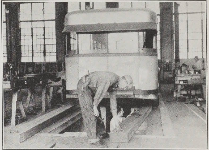
This shows the removal of timber after coach has been run over pit to allow the use of full width of pit.
