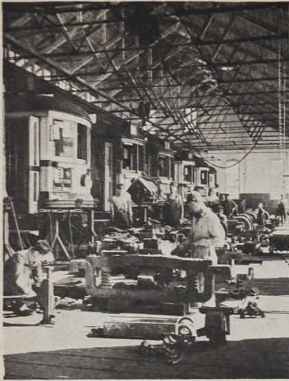
A corner of the Truck Repair Shop
