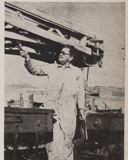
Painter Frank Bache (1919) finishes up on a derrick job.
