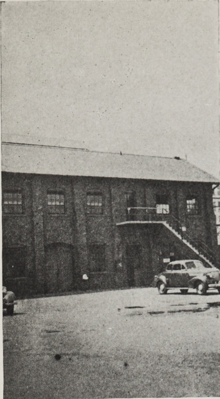
ABOVE—Central Sub-Station, located in the 16th St. Yard. Here also are the offices of Line Dept., Electrical Construction and the Load Dispatcher.
