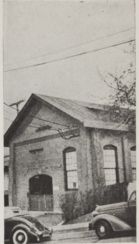
ABOVE — Westlake Sub-Station on Ocean View between Coronado and Parkview.
