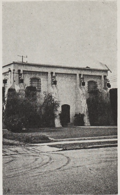
ABOVE — Garvanza Sub-Station. Located at Ave. 56 and Buchanan Sts.
