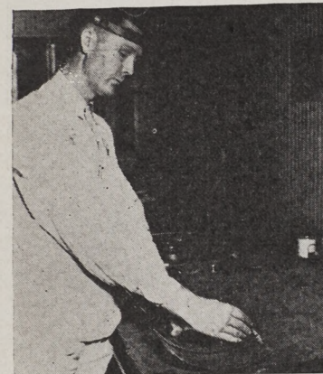
W. Farris cutting glass for corner curved sash.
