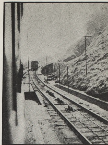
CABLES pull the trains over the steep grades in the coffee country.
