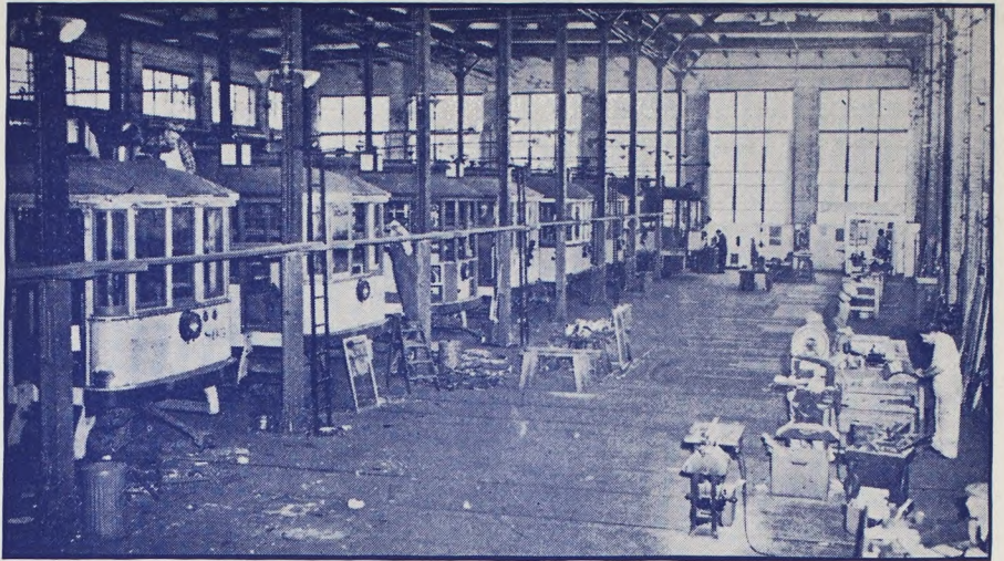
A veritable beehive is the South Park Shops in their new reclamation project. It is quite a sight to see those cars which have been out of service, revamped, refloored, reroofed, repainted until they shine like a Christmas ornament.
