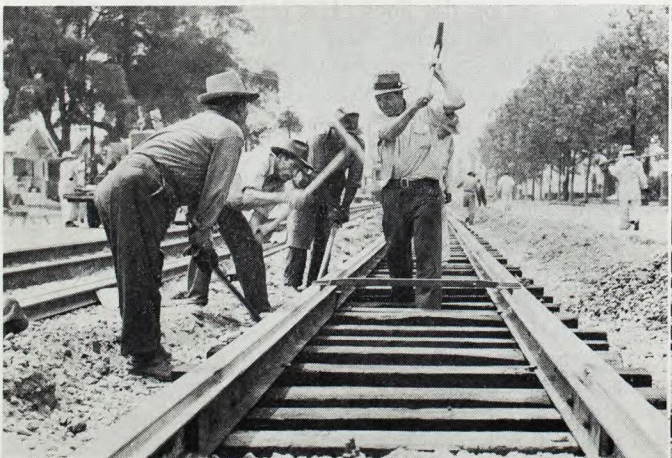
• Rails are spiked to every fifth tie and after this operation cars begin operation.
