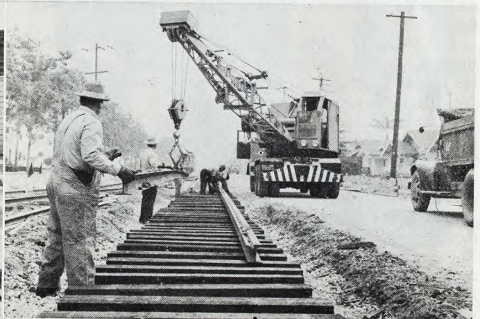
• Rails are laid on the ties with this huge crane operated by Dick Turbeville. • Final step is the pouring of concrete shown below.
