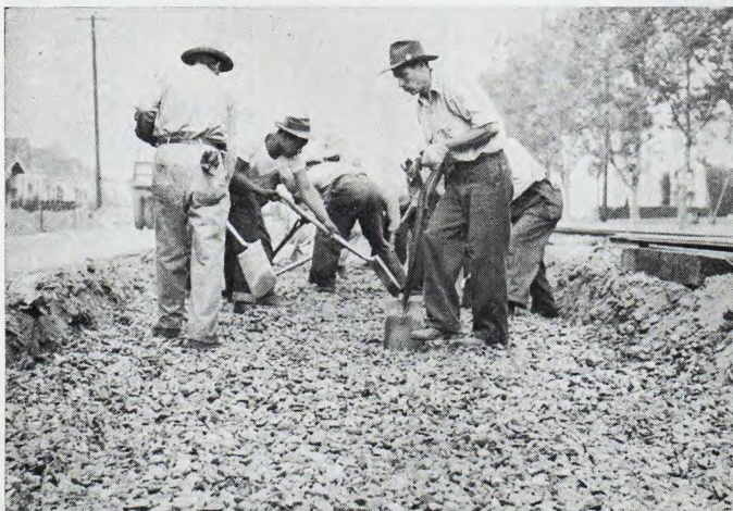
• Below, crews leveling the gravel by hand preparatory to its first rolling.
