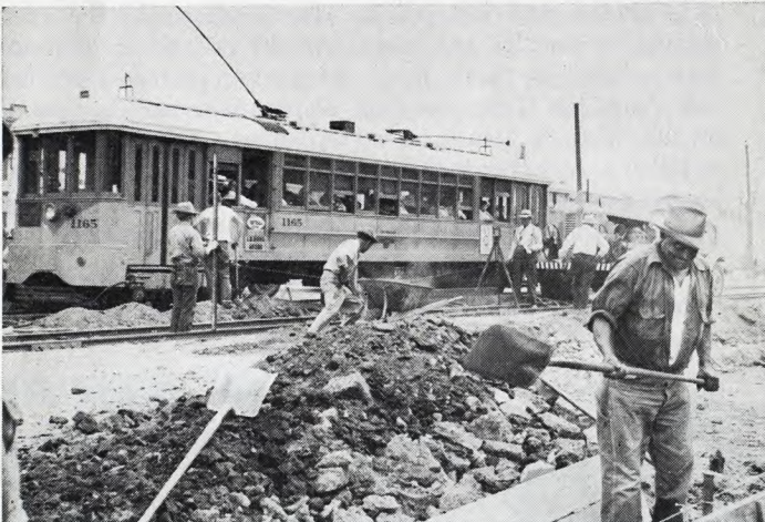
• Below, crews leveling the gravel by hand preparatory to its first rolling.
