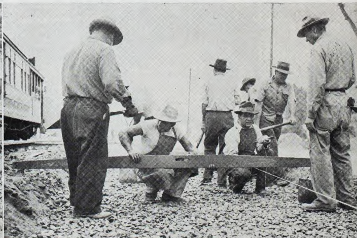
• After gravel is rolled more gravel is thrown on top and a worker with a level checks the grade.
