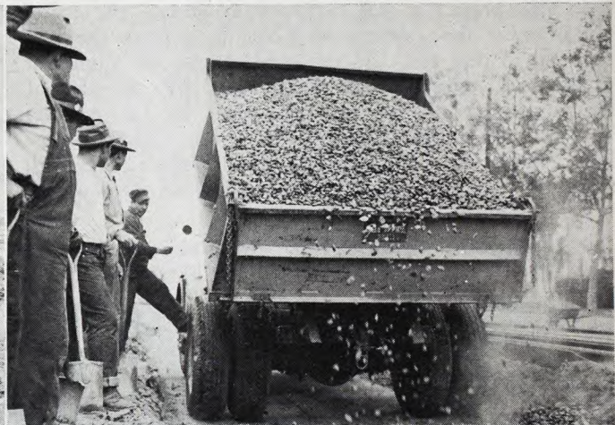
• After gravel is rolled more gravel is thrown on top and a worker with a level checks the grade.
