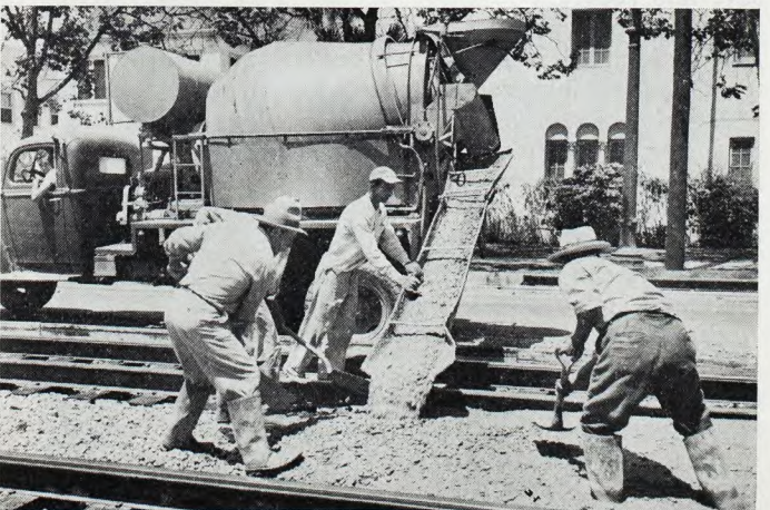
• Rails are laid on the ties with this huge crane operated by Dick Turbeville. • Final step is the pouring of concrete shown below.
