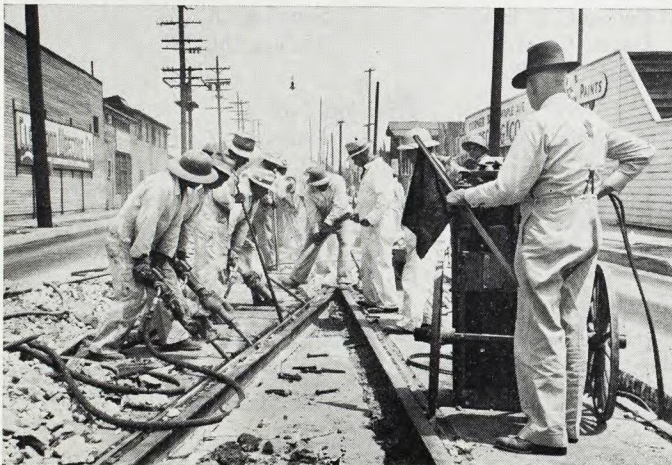
• Rails are spiked to every fifth tie and after this operation cars begin operation.
