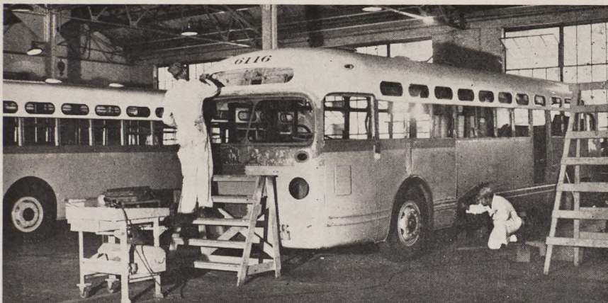
Busy view of the Body Shop at 16th Street Garage showing two coaches in the rebuilding process; one on the left has been finished, the other stripped down to its skeleton is having panels added preparatory to a complete sanding and paint job.
