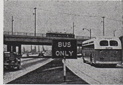
When Bus operation begins on Freeways express busses or "Freeway Flyers" will enter bus turnouts, where patrons may board or leave the vehicles via specially built loading platforms, well out of the stream of motor traffic.
