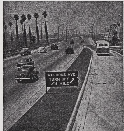
The "Freeway Flyer" emerges from bus turnout into right lane of Freeway. This shows the ease with which mass transit vehicles can re-enter the traffic lanes without impeding traffic.
