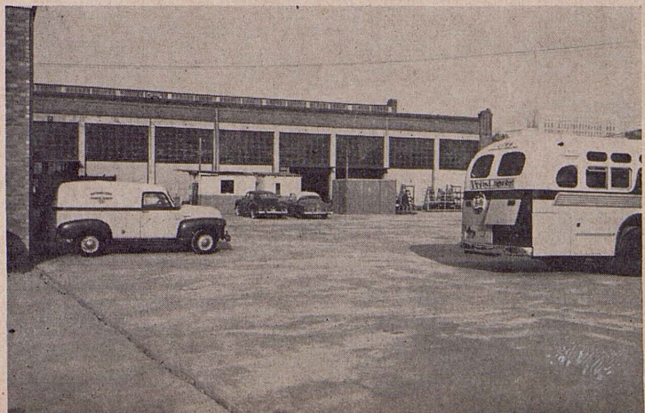
New paving around repair shop. (Not all is shown in this photo.)
