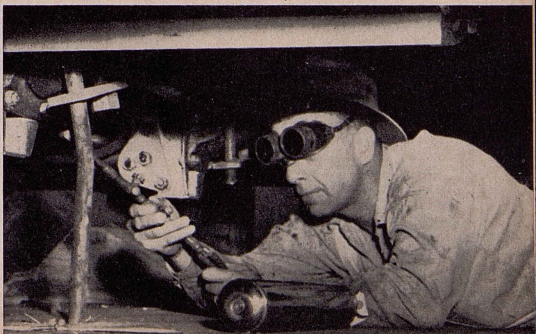
7. CUTTING TORCH is applied by Ed Axenty to the iron rods. With blocks and braces removed, bus backs out of box car.
