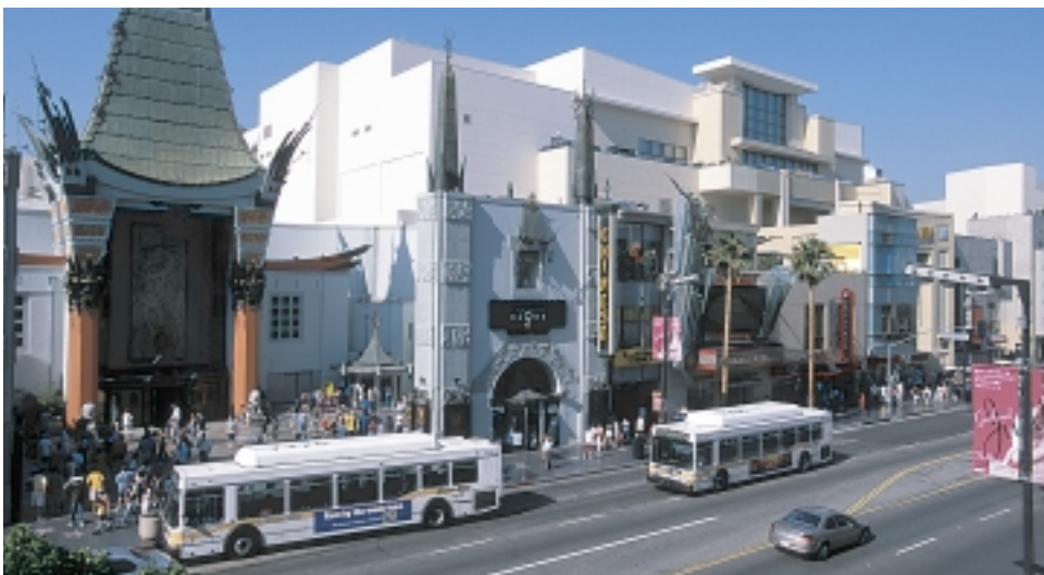
MTA's largest joint development, Hollywood & Highland, is located above the Metro Red Line subway station at the famous intersection. Built next to Grauman's Chinese Theater, the more than 600,000 square foot complex features retail shops, restaurants, general cinemas and the Kodak Theatre, home of the Academy Awards.
