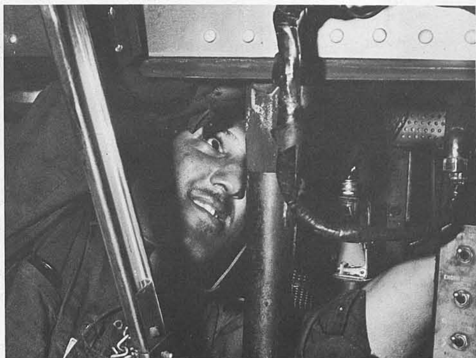
Fletcher Earles, mechanic "B," rewires power box on Bus 5463.
