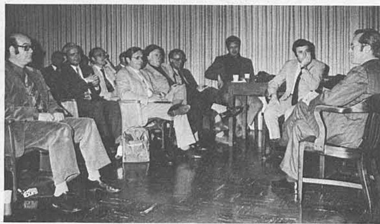
The 24 visiting German transit officials met in the District's Boardroom for a briefing from RTD's General Manager Jack R. Gilstrap. The visitors were particularly interested in the District's plans regarding the Busway and Rapid Transit System. They termed the District's plans as "excellent." As part of their tour of the District they traveled by RTD bus along the Busway construction site in the median of the San Bernardino Freeway.
