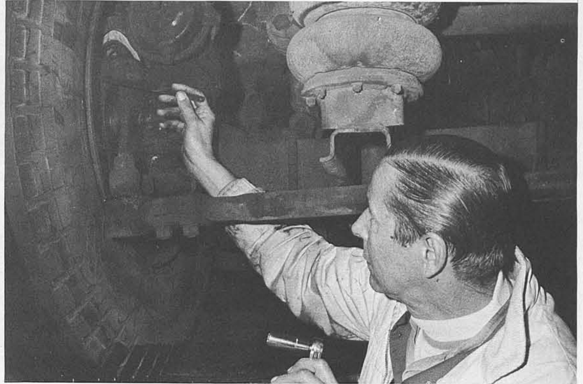
Ed Kennet, Mechanic "A", makes final brake inspection and adjustment before 7049 is given a road test. When 7049 passes its brake test it'll go back to its division.
