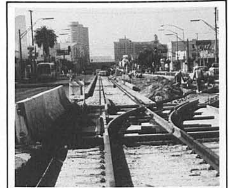
Tracks for the Long Beach-Los Angeles Light Rail Line have been laid along the median of Long Beach Boulevard in the City of Long Beach, as well as throughout most of the mid-corridor section of the route. From Long Beach Boulevard, the route loops around the city's civic center.
