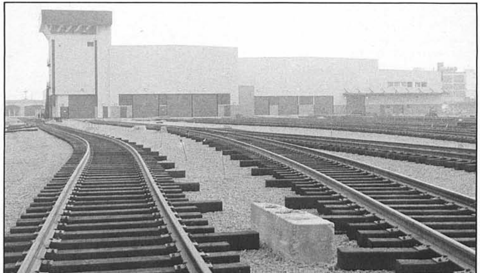
The Metro Red Line communications tower and maintenance of way building just east of downtown Los Angeles near the Los Angeles River is completed.
