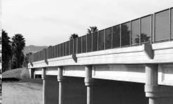
The first of three Metro Orange Line bridges has been completed over the Los Angeles River in the Sepulveda Basin.
