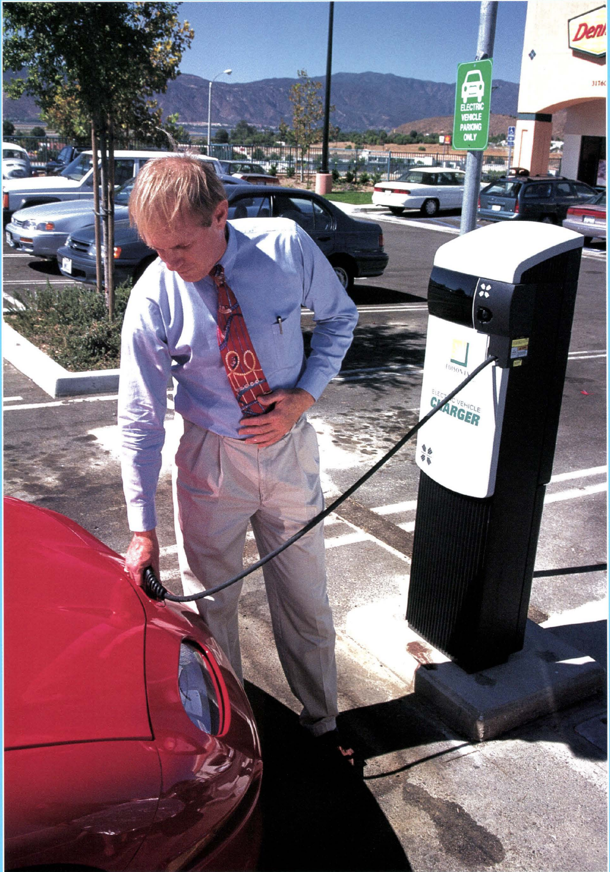
"FILLING UP" ELECTRIC VEHICLES WILL BECOME ROUTINE AS MORE PUBLIC CHARGING STATIONS ARE INSTALLED ACROSS THE SOUTHLAND.
