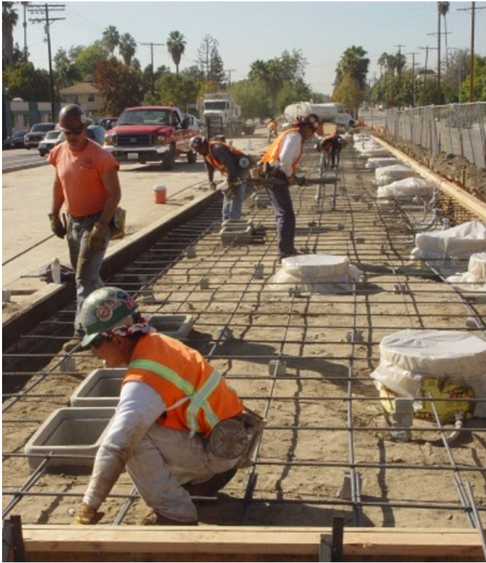
Orange Line -- Forming Platform of Laurel Canyon Station
