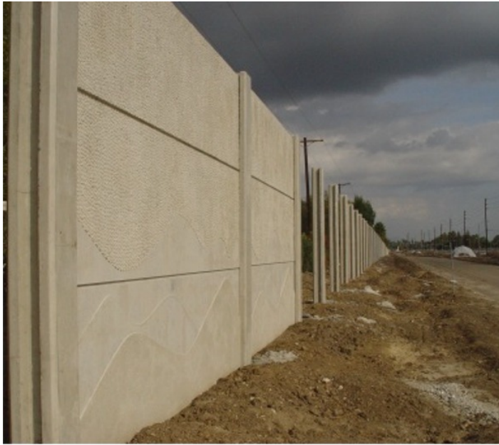
Orange Line -- Sound wall north of Victory Blvd.
