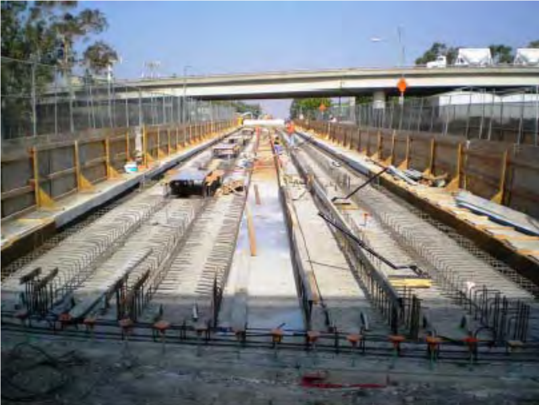
Gold Line Eastside Extension – Construction at I-710 Freeway
