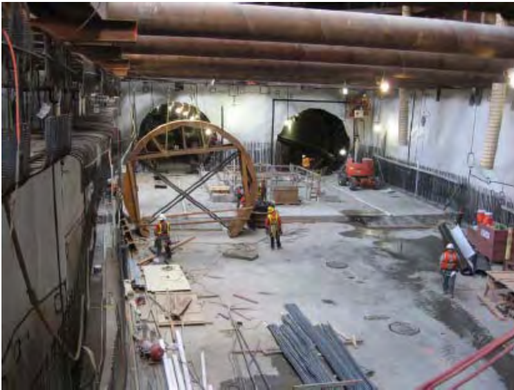
Gold Line Eastside Extension Project – Construction at Soto Station
