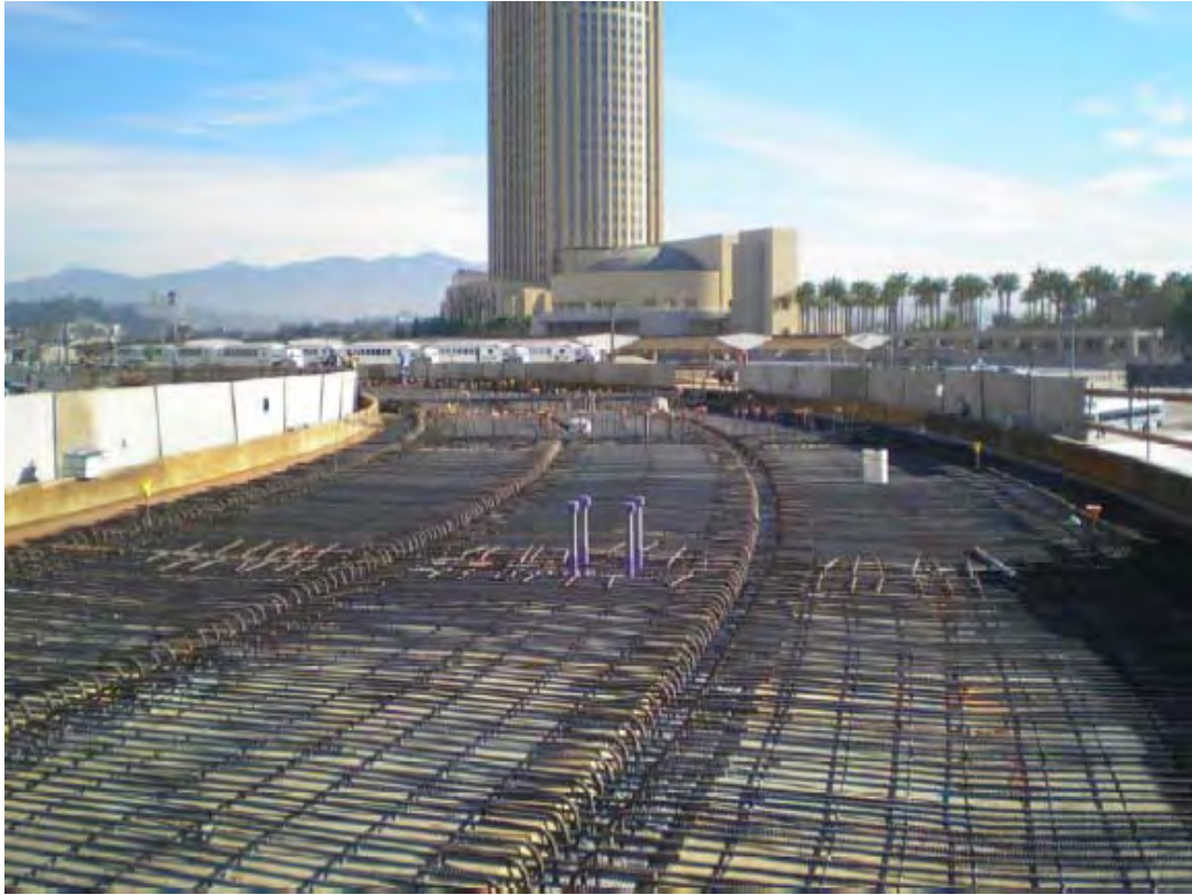
Gold Line Eastside Extension Project – Bridge over 101 Freeway
