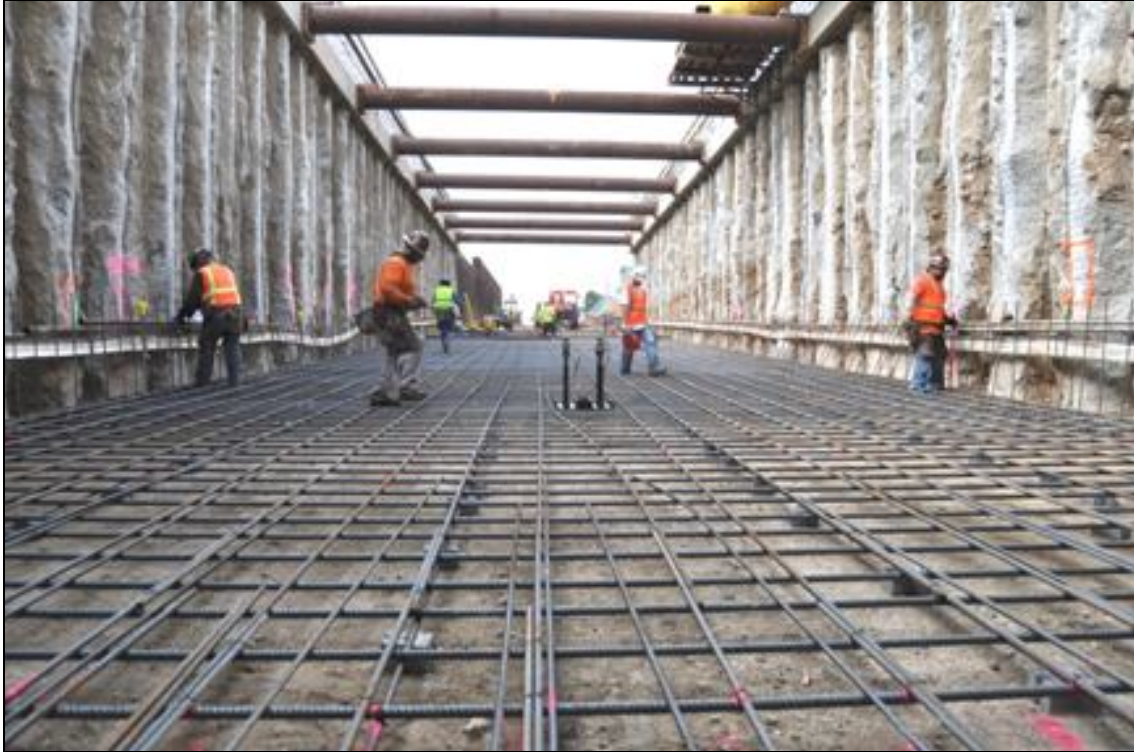
Rebar Work on Trench Slab
