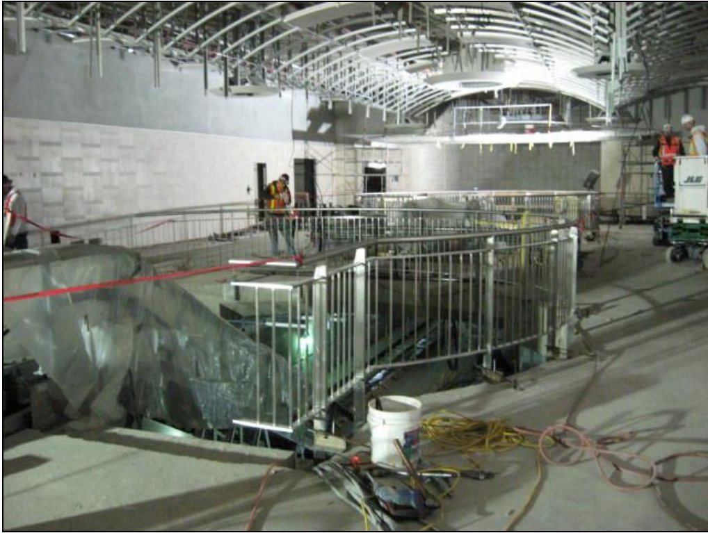
Boyle Heights / Mariachi Plaza Station – Mezzanine Construction
