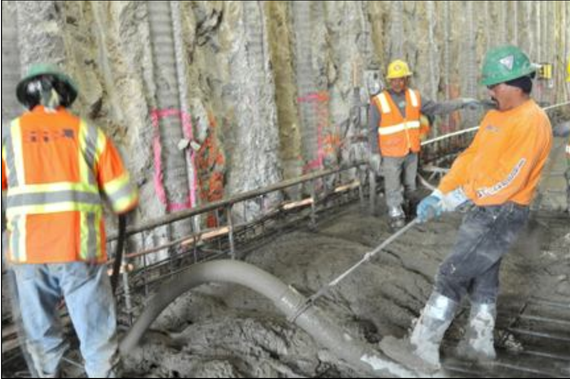
Pouring of Trench Slab
