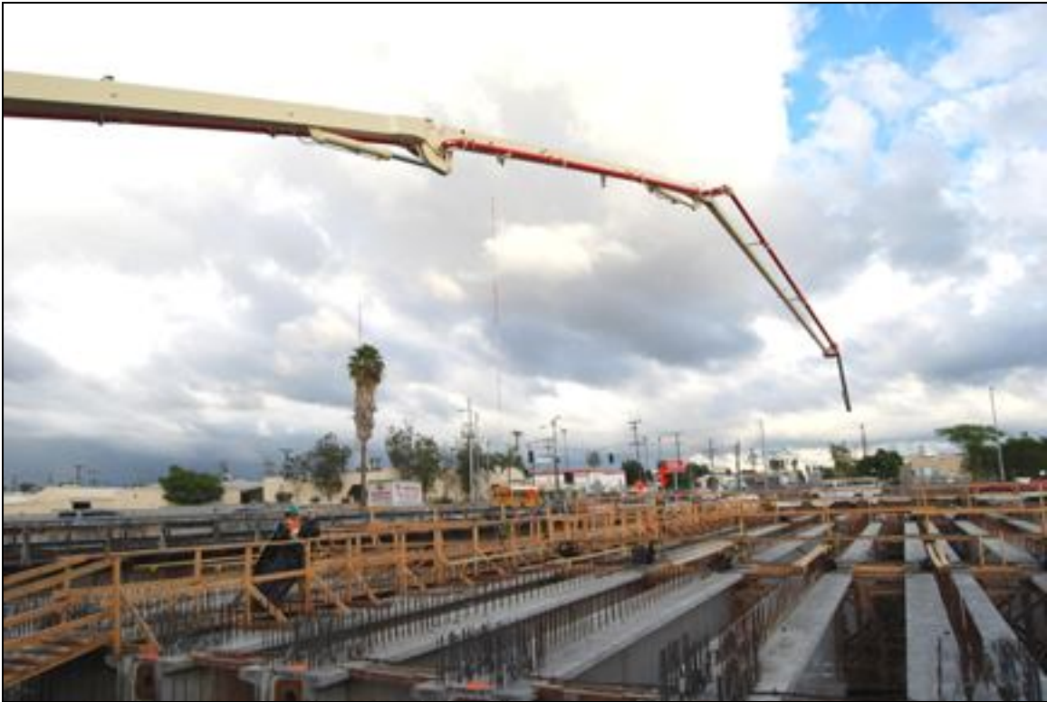
National Bridge Pouring
