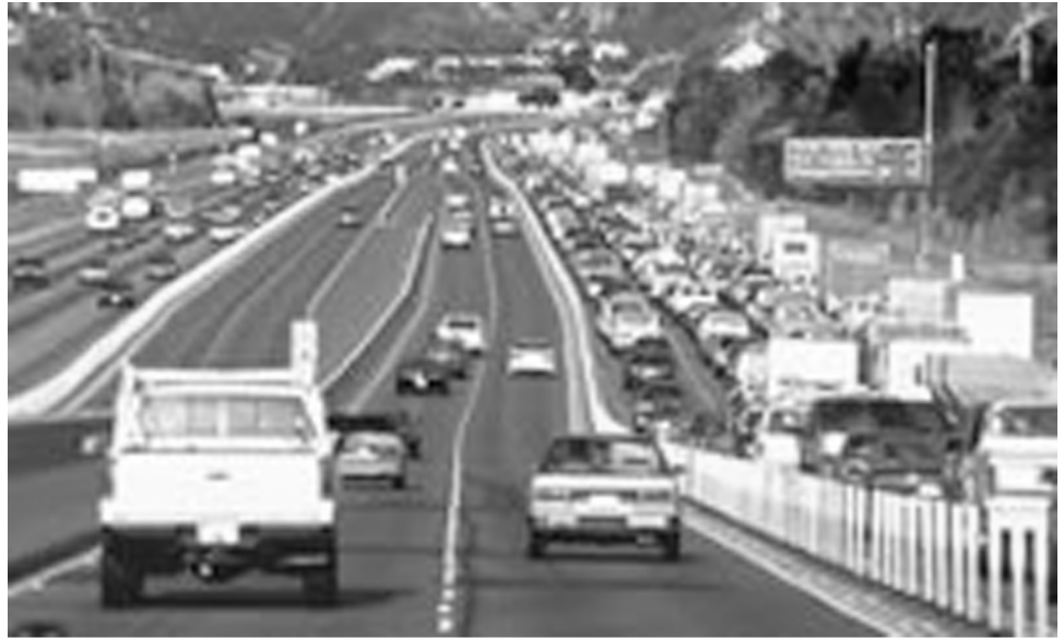
Figure 1: Tolled Lanes on State Route 91 in Orange County, California
