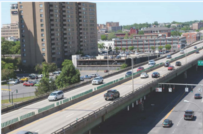
Current: A section of Interstate 81 on a viaduct that runs through Syracuse, New York.
