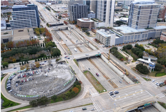
Before: A section of the Woodall Rodgers Freeway, before being capped.
