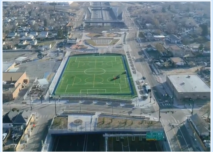
After: The same section of land with a cap park and sports fields built over Interstate 70.
