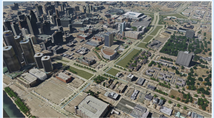
Planned: The planned removal would allow for a boulevard and additional acres of land for redevelopment.
