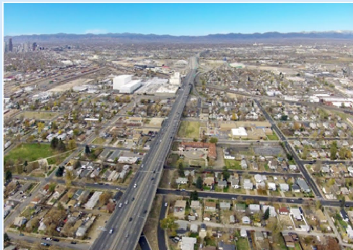
Before: A section of Interstate 70, before being capped.
