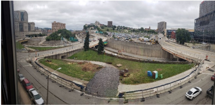
Before: A section of Interstate 579, before being capped.
