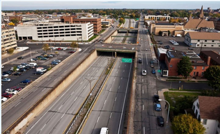
Before: The eastern segment of the Inner Loop before removal.
