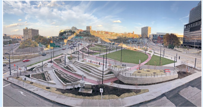
After: The same section of land with a cap park built over Interstate 579.
