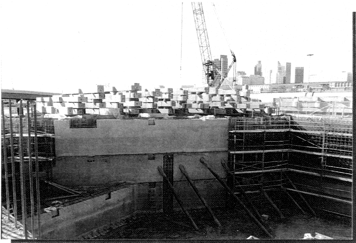
PUBLIC TRANSIT PARKING – LOOKING SOUTH SHORING – SHOTCRETE WALLS – PRECAST COLUMN STORAGE
