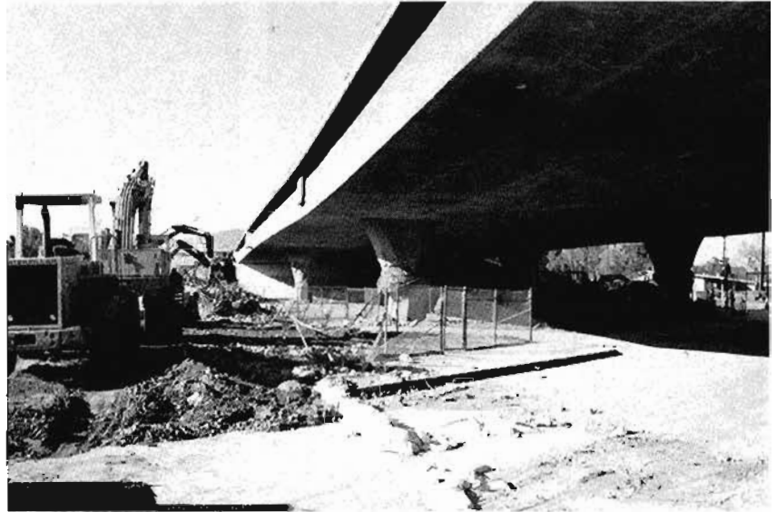
Figure 3-7. Flexure/shear failure in the bottom of the flared columns still visible in the westbound bridge, even though demolition was in full progress at the SR-118 Mission & Gothic Undercrossing. (photo: F. Seible)
