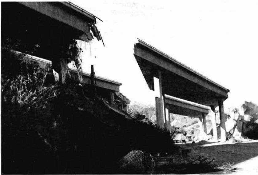
Figure 4-1. I-5, Gavin Canyon Undercrossing, Northridge earthquake. (photo: F. Seible)
