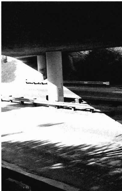
Figure 3-6. Columns retrofitted with circular steel jackets at the Cadillac Avenue offramp directly adjacent to Washington and Fairfax. These columns survived without problems the same ground accelerations that caused the Washington and Fairfax collapse (Figures 3-4 and 3-5). (photo: F. Seible)
