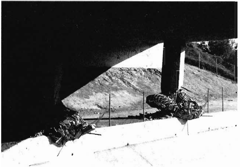
Figure 4-8. Bull Creek Canyon Channel Undercrossing, SR-118, Northridge earthquake. (photo: T Saido)
