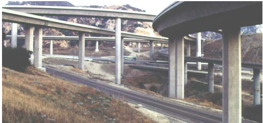
Figure 7-19. Reconstructed I-5 interchange.
