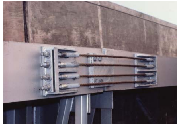
Figure 9-2. External cable restrainer.
