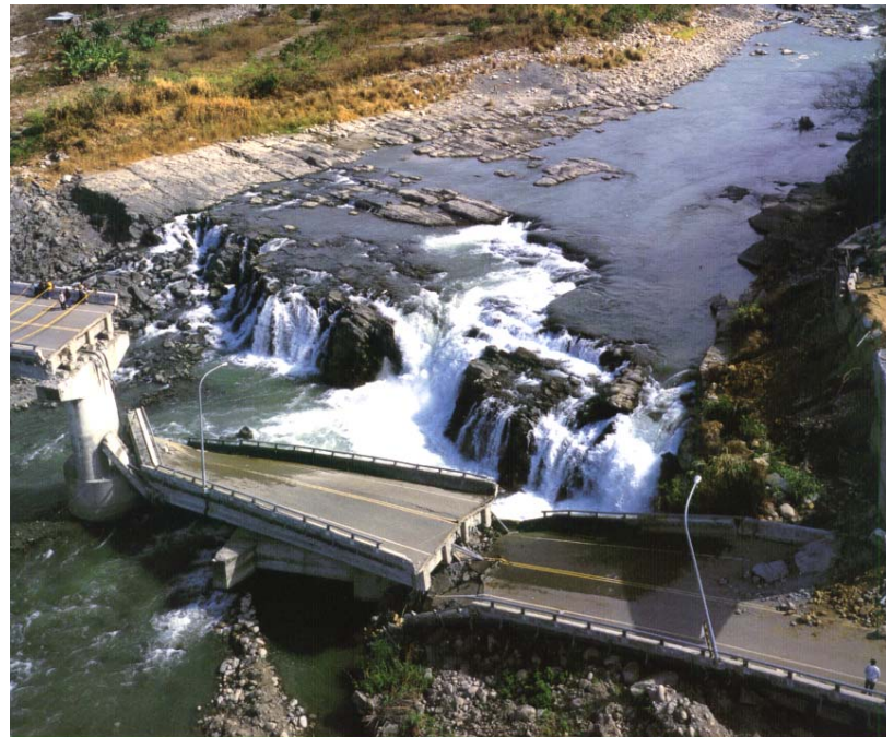
Figure 5-4. The Chelungpu fault scarp as it crosses the Tachaihsi River, producing a 6-meter-high waterfall and destroying the road bridge. The damaged Shihkang dam is in the distance (from Bolt 2003; photo courtesy of Jack Un, Flying Tiger Photographic, Inc.).
