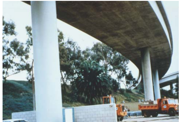
Figure 7-10. Good performance of new column retrofit detail.
