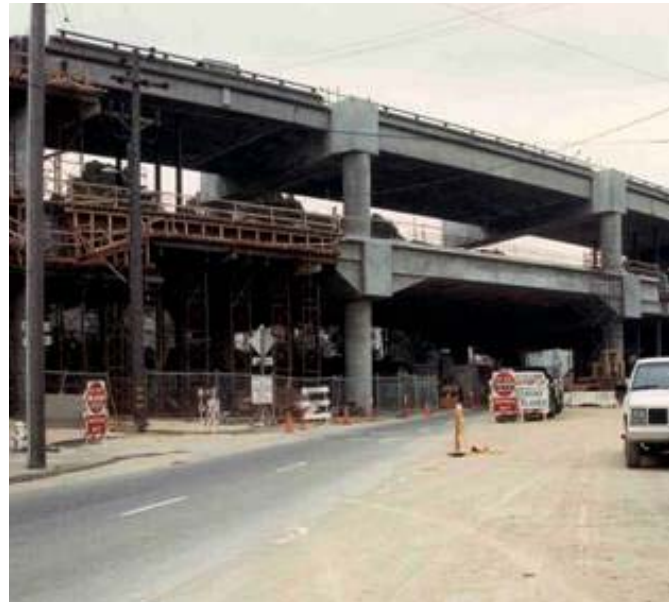
Figure 9-10. San Francisco double-deck viaduct retrofit.
