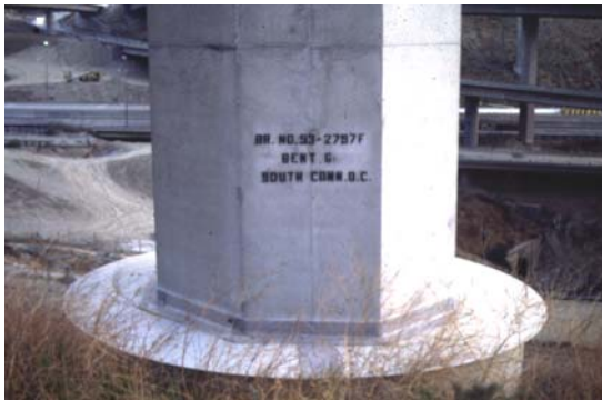
Figure 7-21. Isolation casing for short columns.
