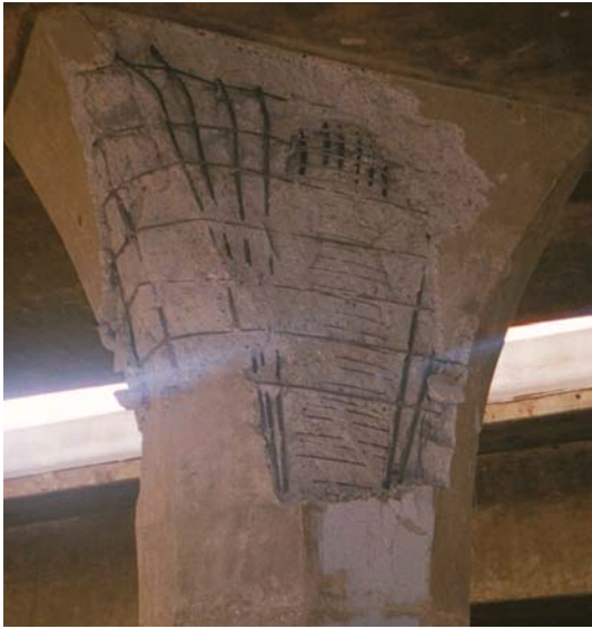
Figure 7-24. Expected performance of column architectural features.
