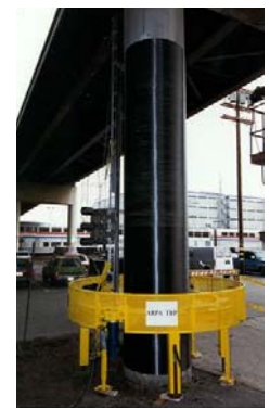
Figure 9-18. Carbon fiber jacking of bridge columns.
