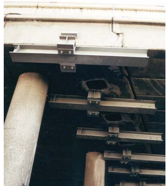
Figure 9-3. Seat width problems and seat extensions.
