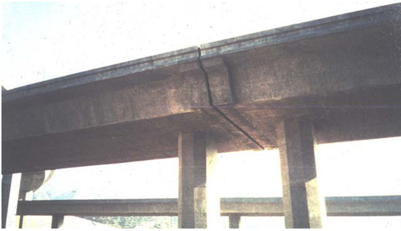
Figure 7-20. Special hinge for large displacements.
