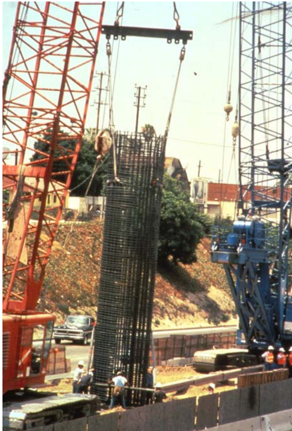
Figure 7-9. New column reinforcing.
