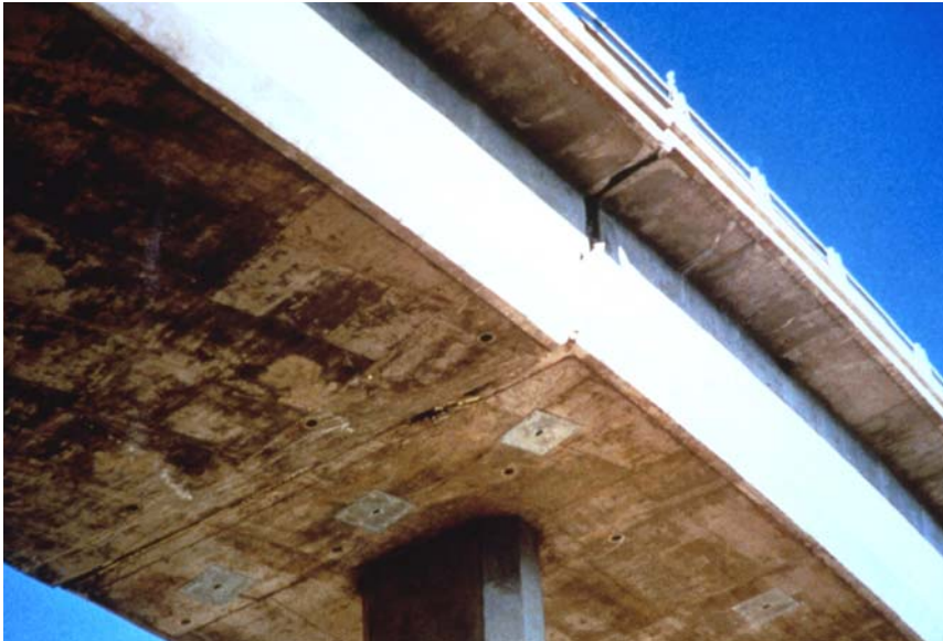
Figure 7-8. Good performance of new hinge restrainer detail.
