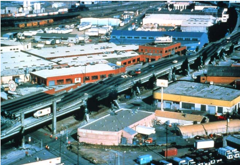
Figure 7-12. Cypress Street Viaduct collapse in Oakland during the 1989 Loma Prieta earthquake.
