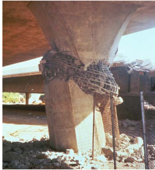
Figure 7-25. Actual performance of flared column.
