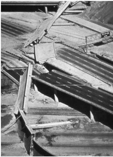
Figure 7-2. Separation of thermal expansion joints.
