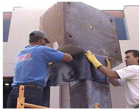
Figure 9-17. Seismic retrofit of a masonry building using wet lay-up of fiber reinforced polymer (FRP) jackets for column retrofit.
