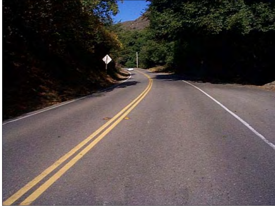
Figure 3.3 PCI = 98 (Excellent Condition)
